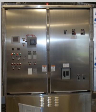
Triplex Pump Control Panel
