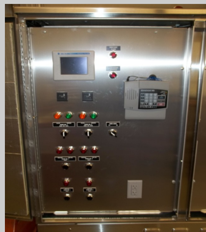
Duplex Pump Control Panel
